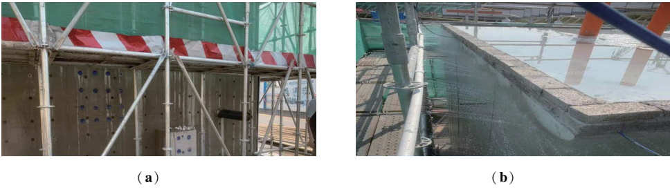
图 4 侧面养护 Fig. 4 Curing condition of side
